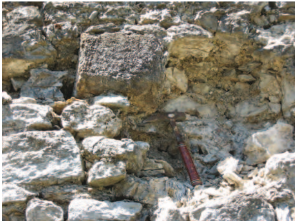
Slika 9.15: Blok oligocenskega konglomerata (OK) v notranjem zidu. Figure 9.15: A block of Oligocene conglomerate (OK) in the inner wall.
