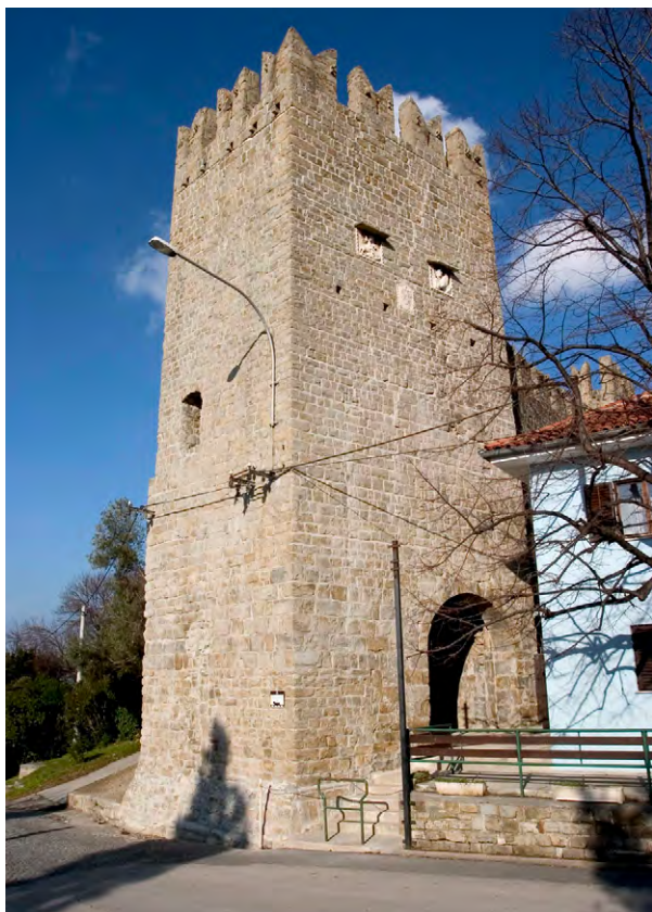
Slika/Figure 9 Stolp 5, vrata sv. Nikolaja (foto E. Lažar, arhiv ZVKDS OE Piran). / Wall tower 5, St Nicholas' Gate (photo by E. Lažar, Archive IPCHS Regional Office Piran).
