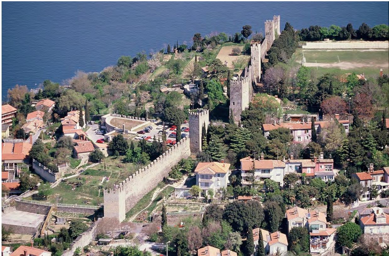
Slika/Figure 1 Srednjeveško mestno obzidje na območju Mogorona, postavljeno v letih 1470–1533 (foto J. Jeraša, arhiv ZVKDS OE Piran). / Medieval town walls in the area of Mogorona Hill, constructed between 1470 and 1533 (photo by J. Jeraša, Archive IPCHS Regional Office Piran).
