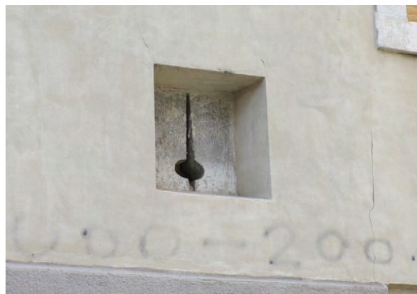
Figure/Slika 13 Inverted keyhole embrasure (loophole), 12 Supilova ulica, 2018 (photo by P. Karković Takalić). / Ključasta strelnica na Supilovi ulici 12, 2018 (foto P. Karković Takalić).
