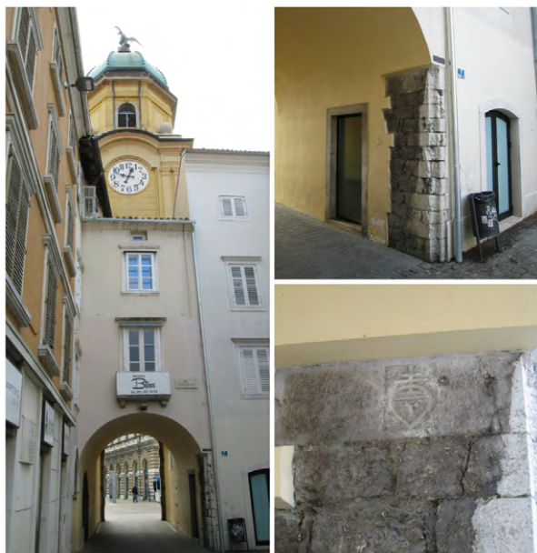
Figure/Slika 15 Clock Tower with remains of a late medieval city gate and late Gothic stonemason's mark (photo by P. Karković Takalić). / Stolp s uro s ostanki poznosrednjeveških mestnih vrat in s poznogotskim kamnoseškim znakom (foto P. Karković Takalić).
