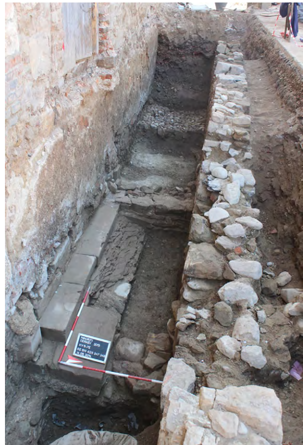
Slika/ Figure 13 Odkrito stopnišče vhoda v gotsko cerkev na zunanji strani ob severni steni cerkve (foto B. Tušek; arhiv PJP, d. o. o.). / An excavated staircase of the entrance to the Gothic church on the outside along the north wall of the church (photo by B. Tušek; PJP, d. o. o., archive).
