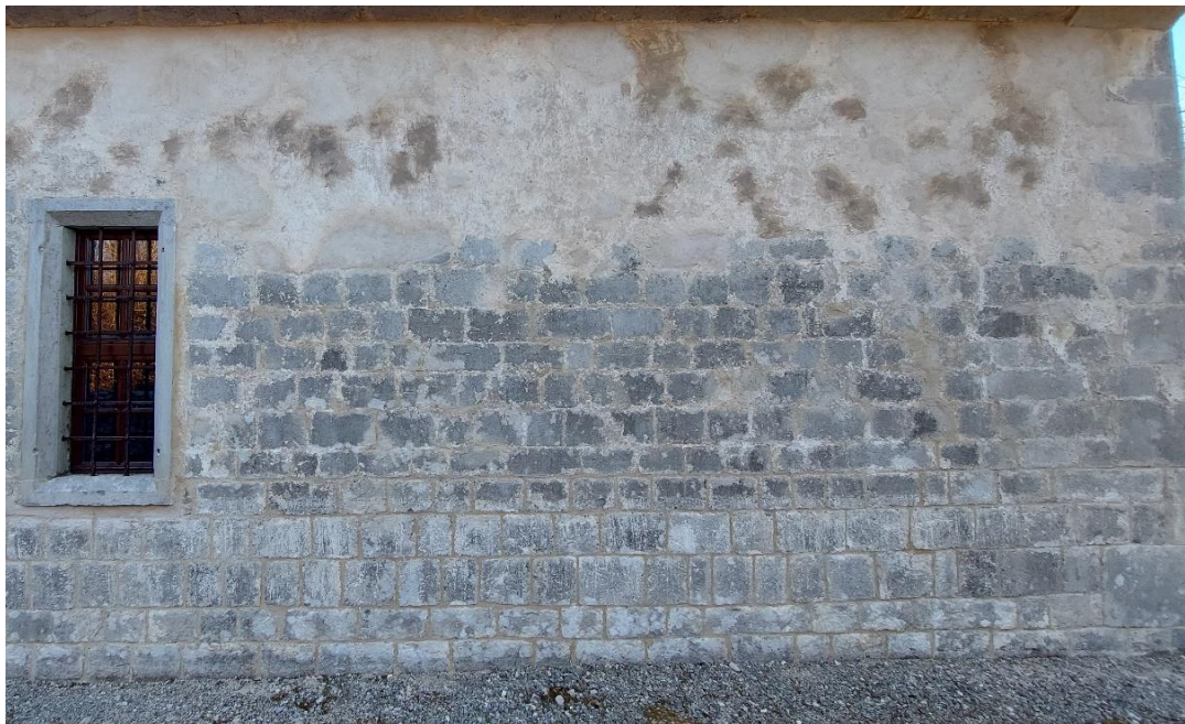
Photo 3: The ashlar masonry on the north wall of the Church of Saint Helen (by: Minka Osojnik).
