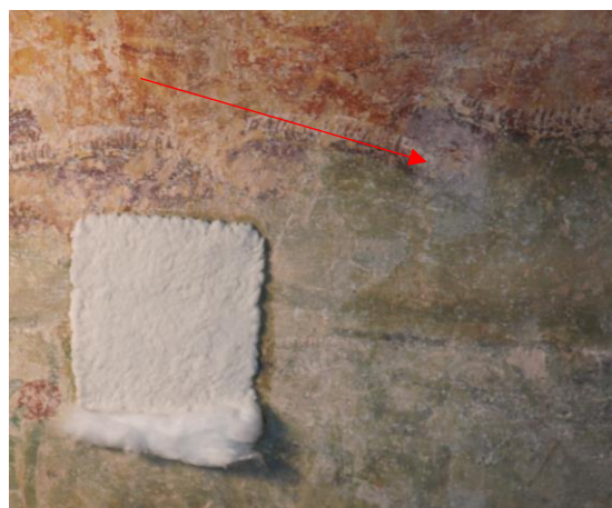
Some whitening after the removal of poultice – it can be removed mechanically or with triammonium citrate.
