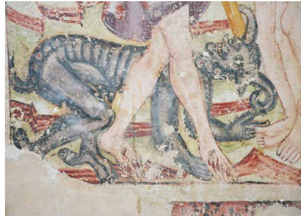
Slika 11: Bele koprne na hudičevem stegnu, ki so se mestoma pojavile po utrjevanju z barijevim hidroksidom (foto: Andrej Jazbec, 2023). Fig. 11: White veils on the devil's thigh which appeared in places after consolidation with barium hydroxide (photo: Andrej Jazbec, 2023).
