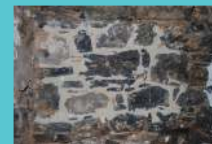
Prefugiranje zidov. Vir: Corradi in sod., 2006
